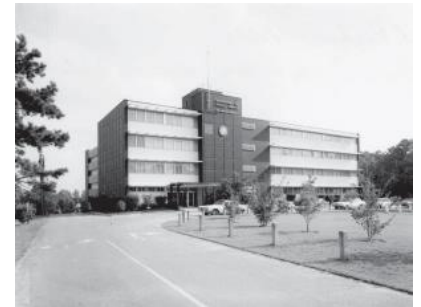
Figure 5. This picture of Neil Kirkman Building was taken in 1969.
