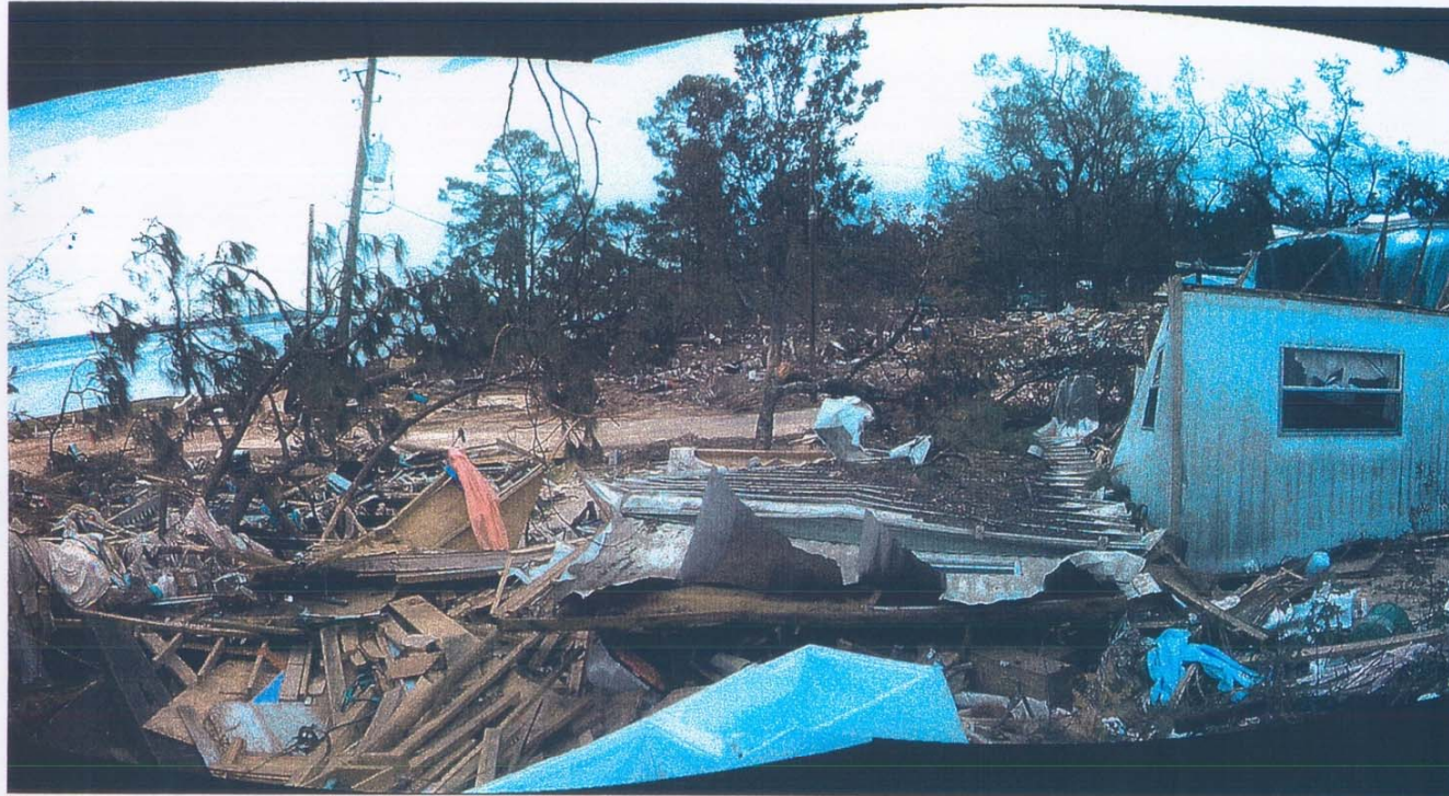
A panorama view of Bay Breeze MHP in Pace. 22 homes in this park and 6 were totally destroyed due to velocity/wave action. All homes were pre HUD and the many straps found on the frames had rusted away from the anchors.
