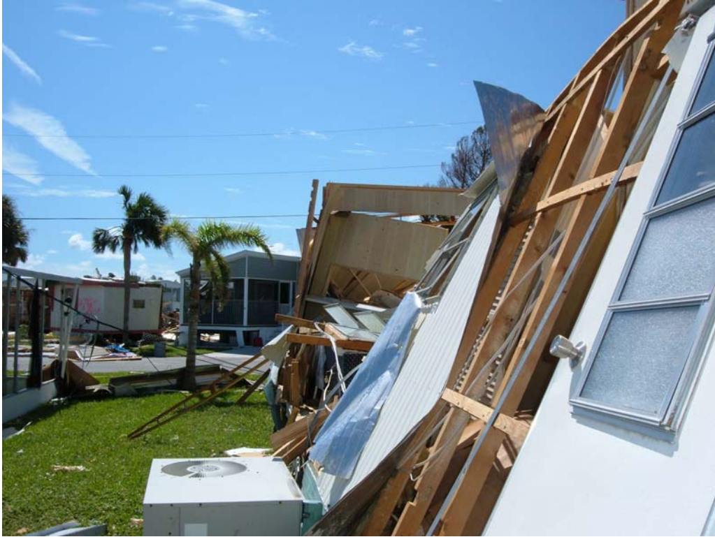
Photographs # 11 through 20 are of the blocking, tie down strap and anchors that show no movement, stress or displacement.
