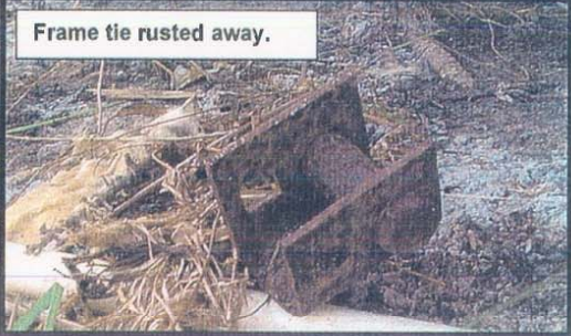
Vertical & frame tie rusted away.
