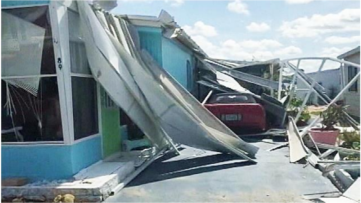
Mobile home s damaged by Hurricane Matthew in Flagler County.
