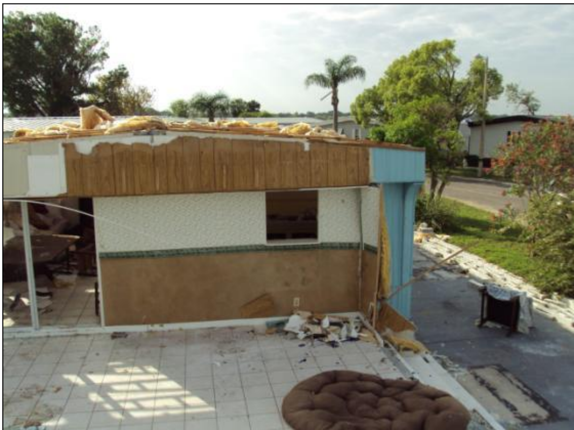
Carport blown away, taking the metal roof off also. The home did not move on its foundation.
