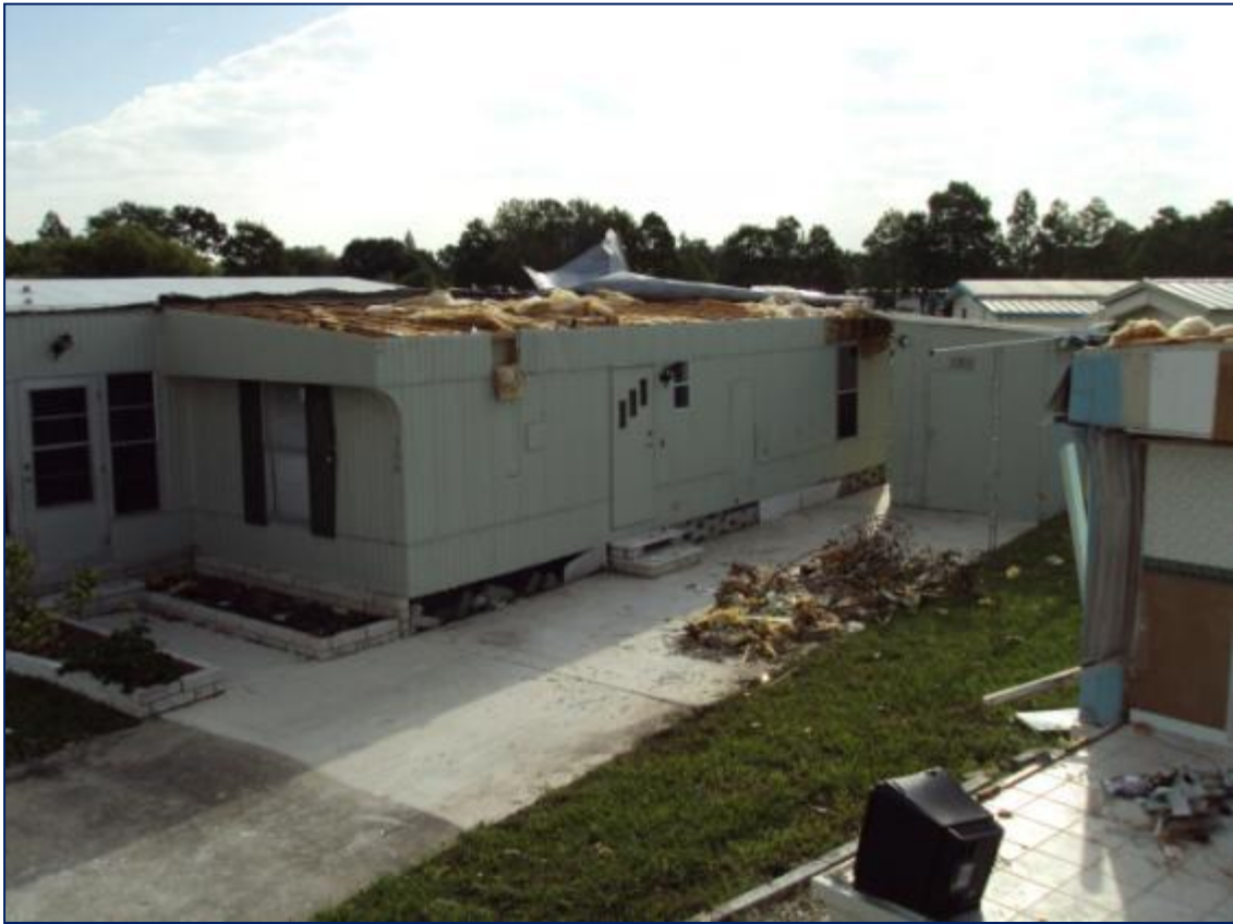
Same home, also missing the front addition which was added after the home was installed.
