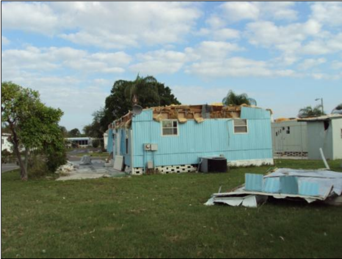
Carport blown away, taking the metal roof off also. The home did not move on its foundation.
