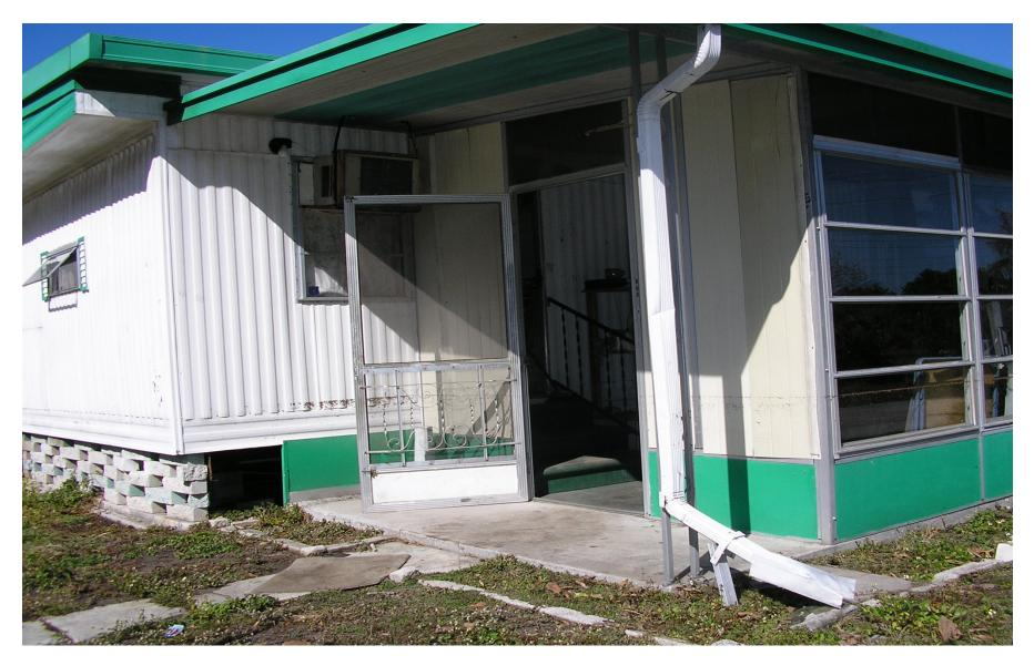
Home on the canal that got 11 ½ inches of water inside. This home is a pre-HUD with 4 over the roof aircraft cables under the skin. The home did not move on its foundation.
