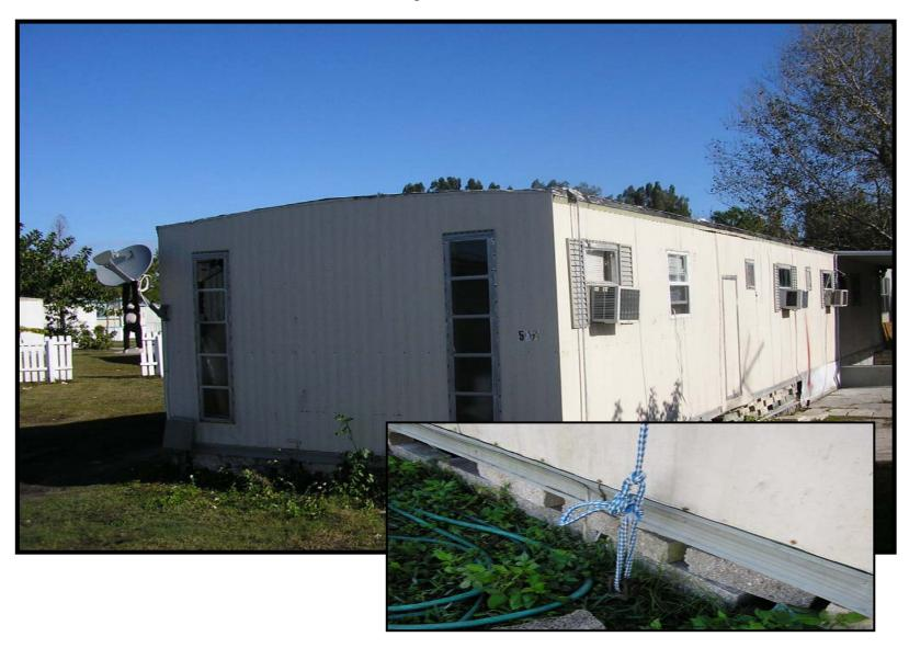
This home is on the canal. The anchor is installed 16 inches out of the ground, however, this home did not move on its foundation. 17 inch debris mark and 10 inches of water inside.
