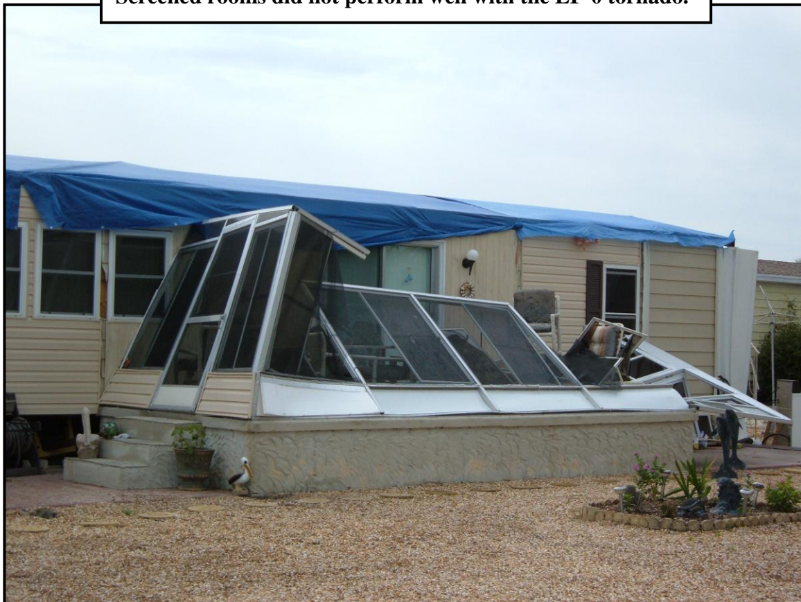
Screened rooms did not perform well with the EF-0 tornado.
